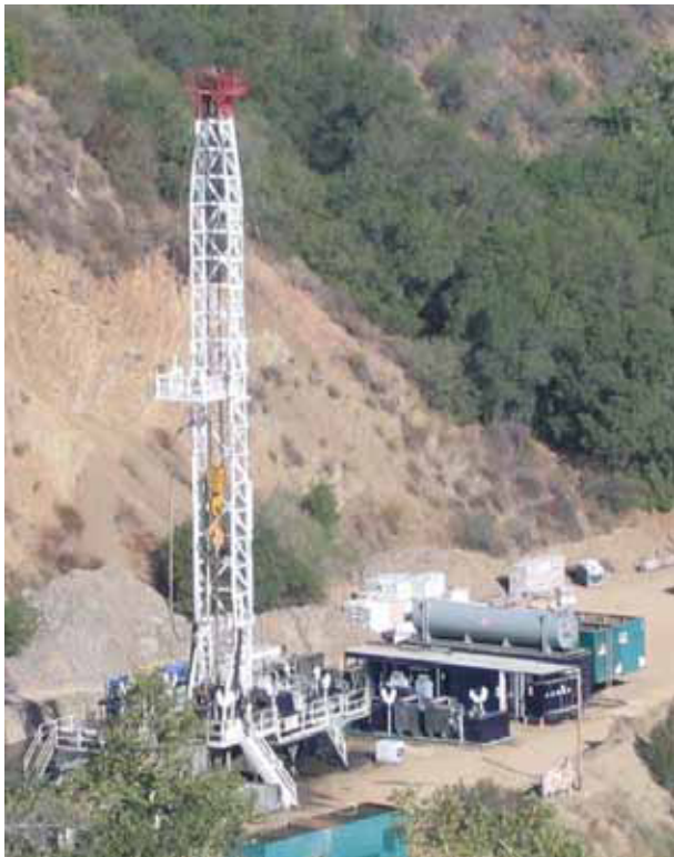
Well Drilling Rig
